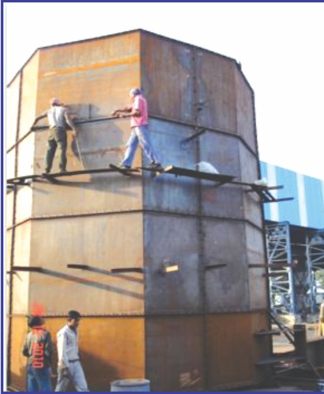
Fig: Main Casing assembly
